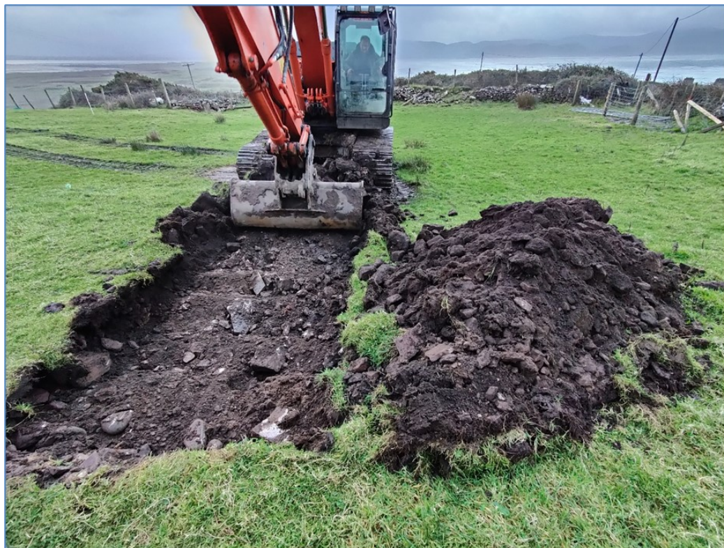
Plate 3: View from north of commencement of test trench T1. Note general context location of nearby ringfort KE045-087 in neighbouring field.
