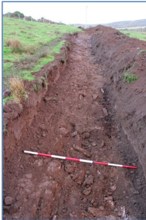
Plate 6: Test trench T14 abutting ZON of KE-045-087 (from SE).
