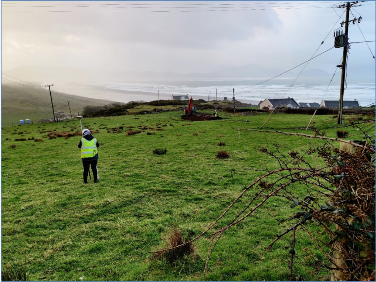
Plate 2: View from north. Excavation of T2 underway. Note myriad overhead power lines.
